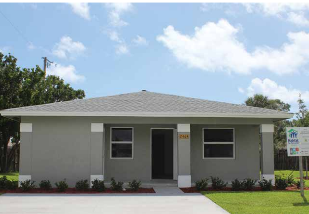
TOP Site plan for A Rick Case Habitat Community ABOVE Habitat for Humanity home on NE 14th Terrace in Pompano Beach
