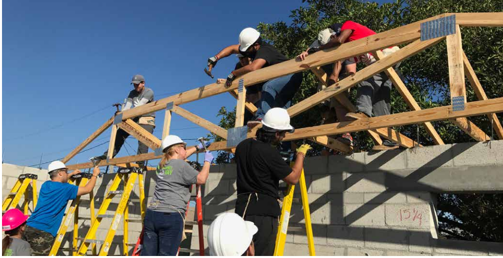
Volunteers work on roof trusses at a Habitat for Humanity home.
